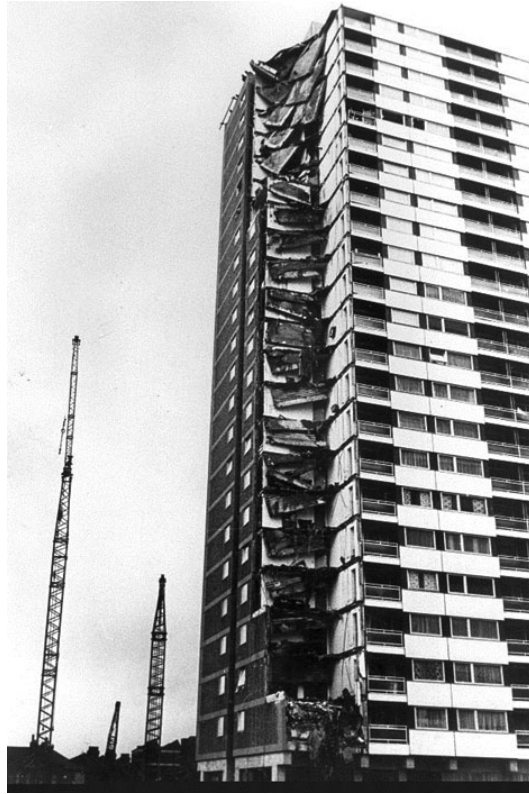
Figure 4: The Ronan Point disaster, 1968 Source: ©London Borough of Newham – Heritage & Archives
