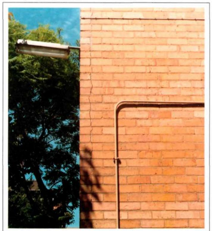
Fig 1 Wall ties have prevented free movement
