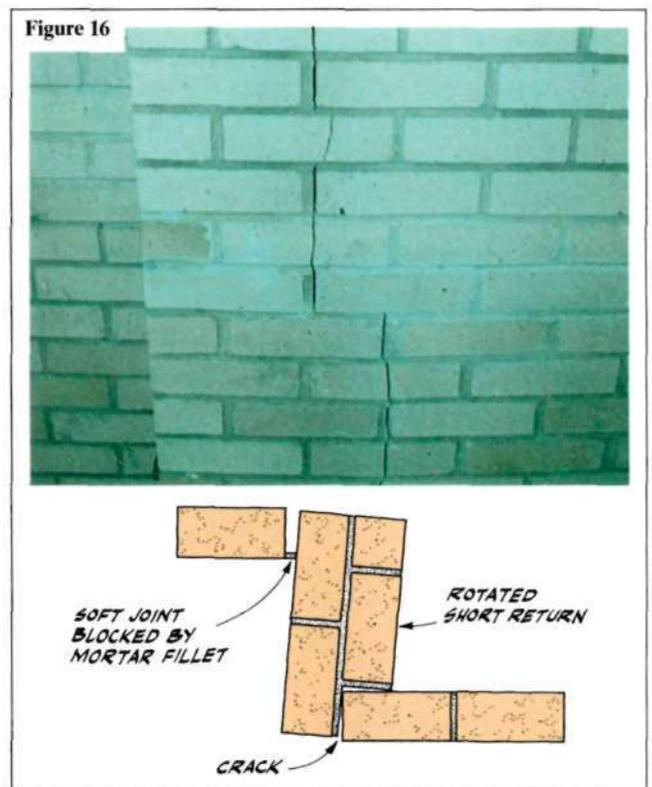
movement joint to allow for any subsequent expansion. In some cases this can be achieved by widening the existing crack but often the brickwork must be restitched and the joint placed elsewhere. The stability of the modified structure must be checked before such work is carried out and additional ties or supports may be necessary.
